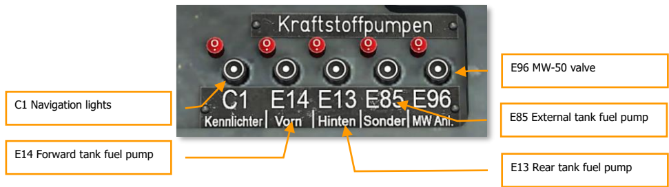
Figure 86: Circuit breakers of additional panel
